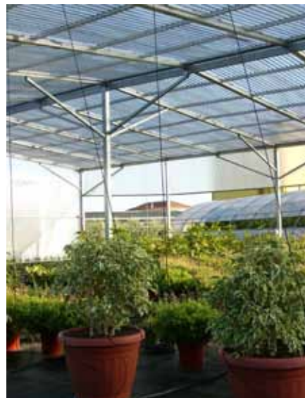
Solyndra greenhouse test-site installation, CeRSAA, Albenga, Italy
